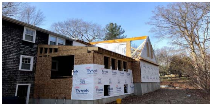
Construction Technology Building Project in Canton by BHR students 2018-2019 school year.
